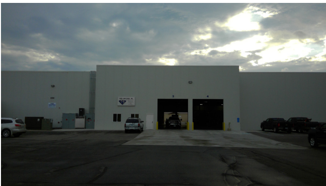
Figure 1: Louis Industries facility, Paynesville, Minnesota
